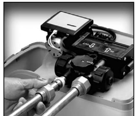
Figure 6: Connect Water Lines
